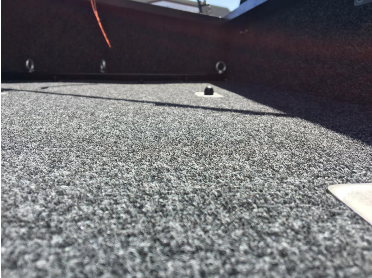
Figure 14: Completed Roof Box Securely Fastened
